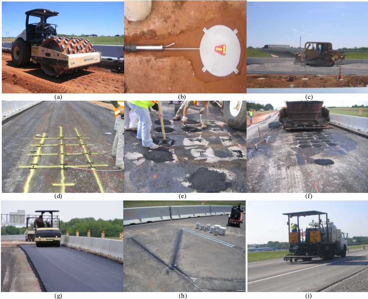
Figure 4: Construction and Instrumentation of Test Section
